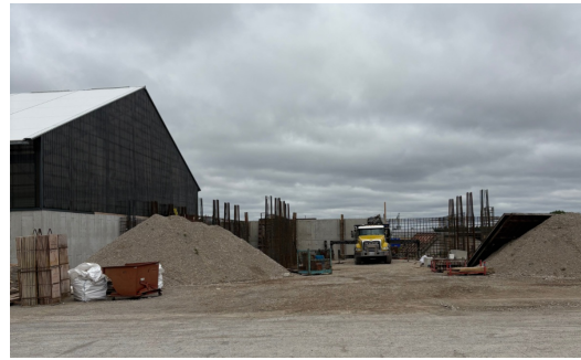
Pictured: Fertilizer tower in the early stages of being built
